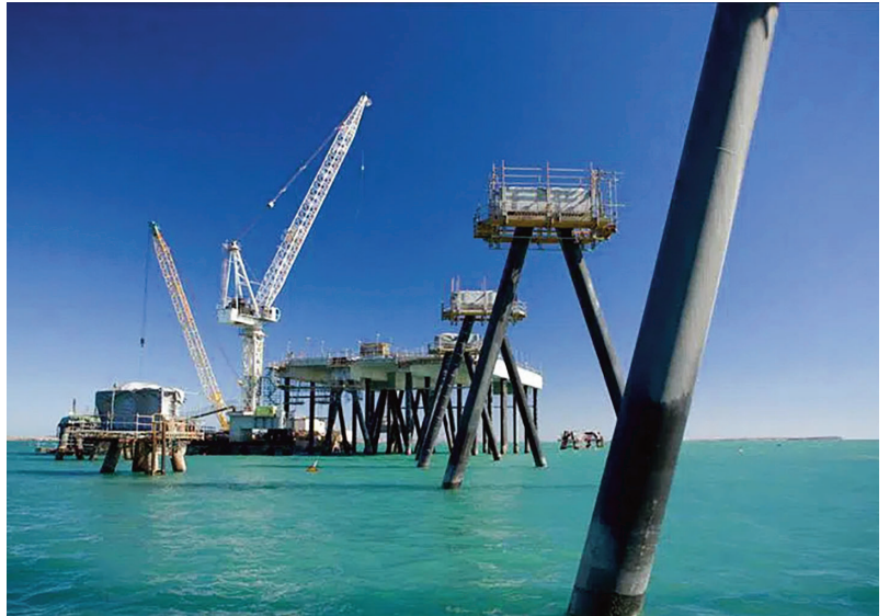
The jetty under construction
