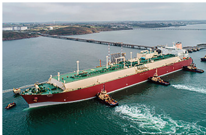
The UK's South Hook import terminal is being upgraded
