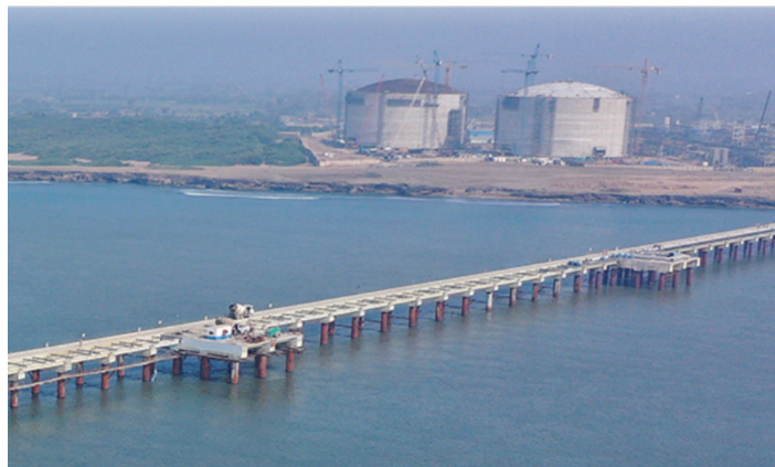
India's newest Chhara LNG terminal located in Gujarat
