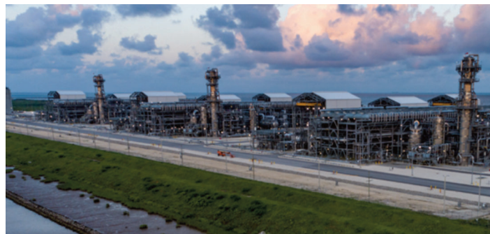
Freeport LNG facility is important part of US export assets
