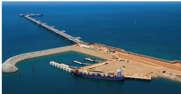
Barrow Island exports facility for Gorgon LNG and products
