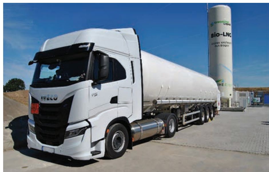
BioLNG truck loading facilities
