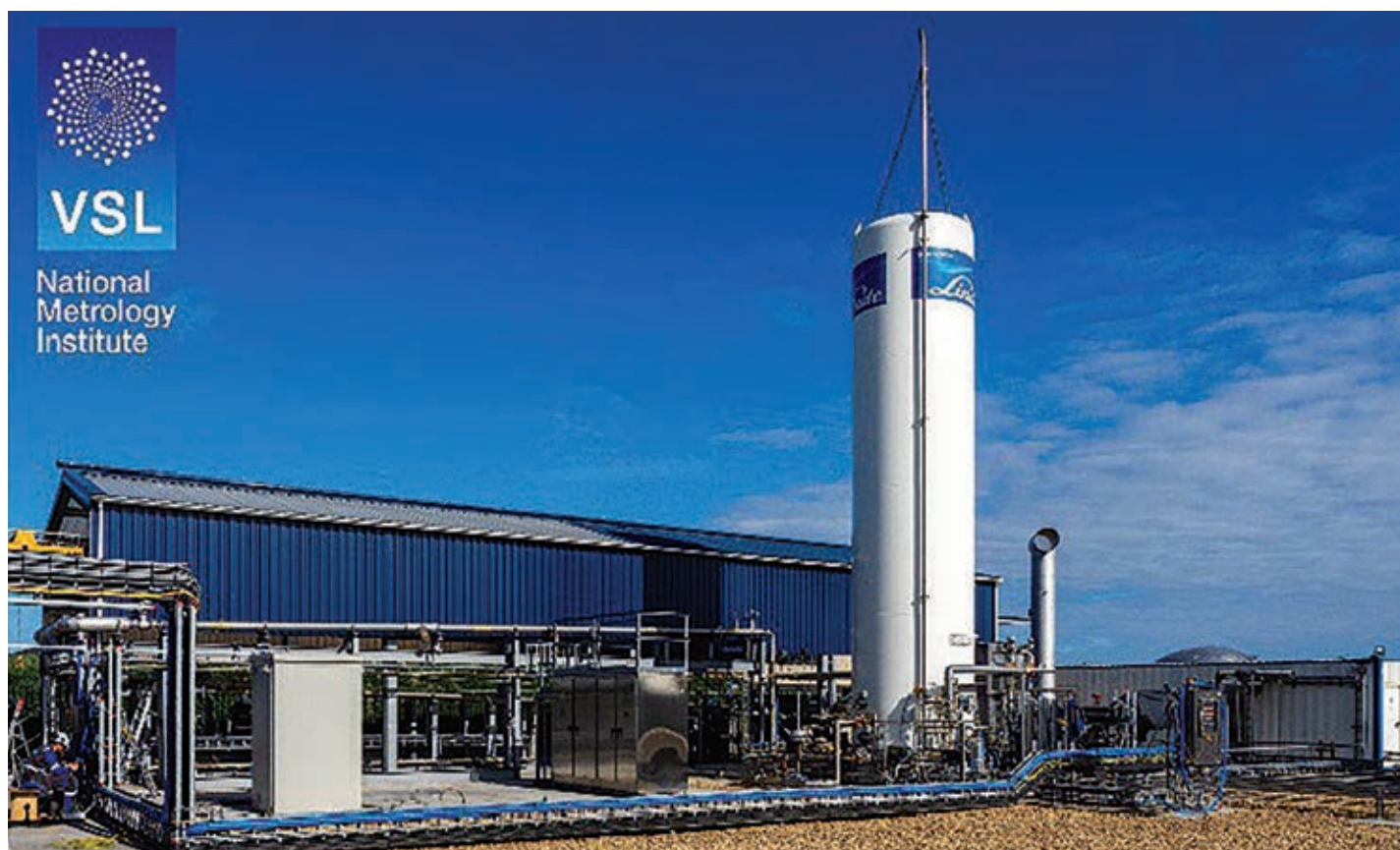
VSL's test facility at Rotterdam's Maasvlakte
