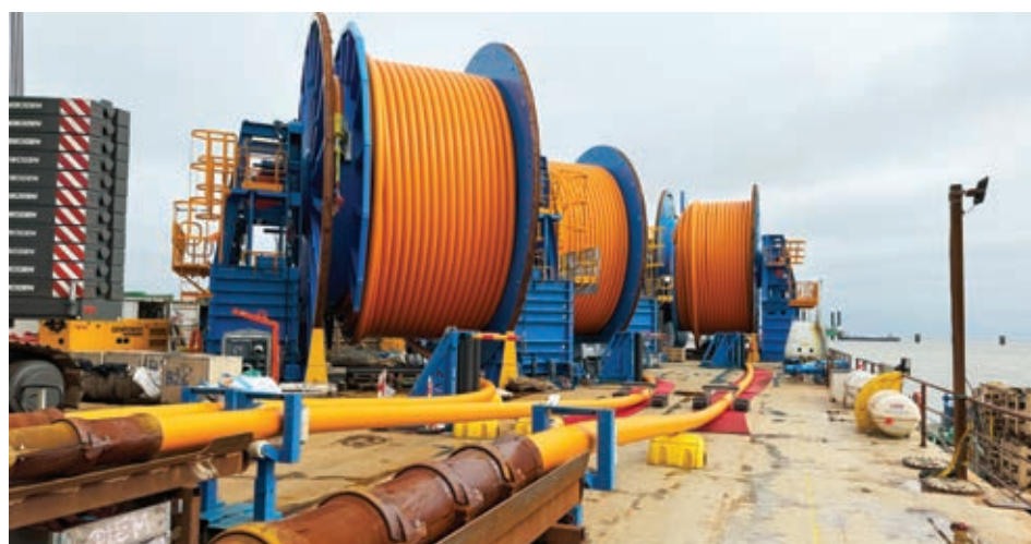
Delivering the pipelines via EConnect's barge
