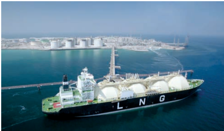
LNG carrier berthing on Das Island in the Persian Gulf
