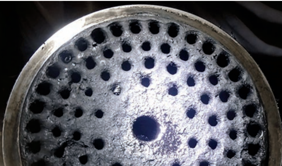
Valve 16-9 viewed by PROGNOST Systems
