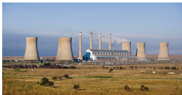
Eskom's Camden power plant
