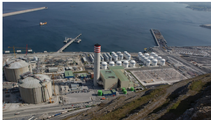
Bahía de Bizkaia Power Station at the port of Bilbao
