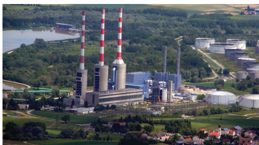
Uniper's 846 MW Irsching power plant
