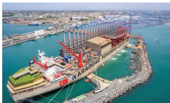
Khan-class Powerships can generate 470 MW on a single vessel
