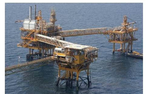
Oil & gas platform at the Mubarek field off Sharjah, UAE
