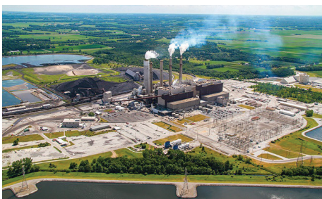
The gas peaker is meant to be built on the R. M. Schahfer site
