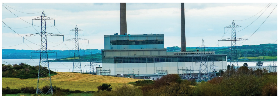
SSE's Tarbert plant in County Kerry
