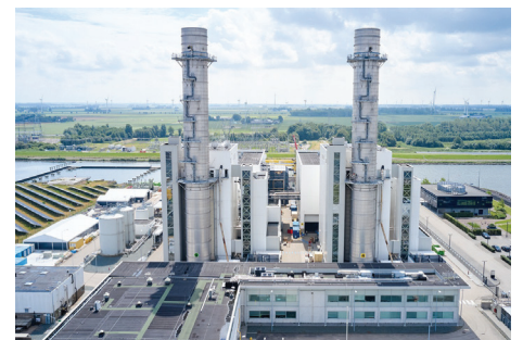
ENGIE's Maxima power plant in Lelystad
