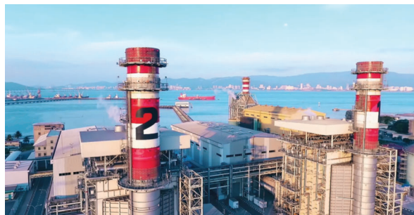
TNB's Prai power station at the coast of Penang
