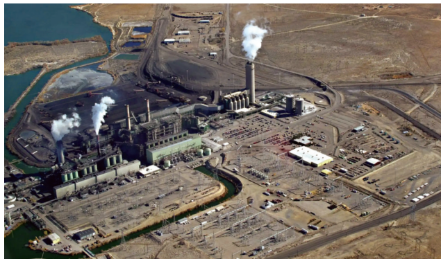
Four Corners power station will not be shuttered early
