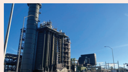
Barry Unit 8 in Mobile County, AL
