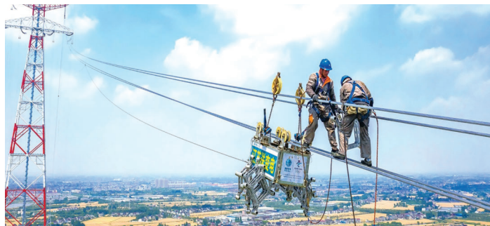
Construction of the 500-kV Yangtze River crossing power line
