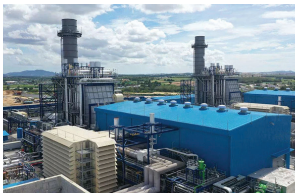
Combined-cycle plant in Rayong
