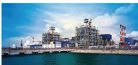
Sakra CHP on Jurong Island
