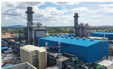
Combined-cycle plant in Rayong
