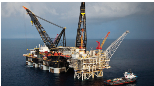
Rig at Tamar gas field
