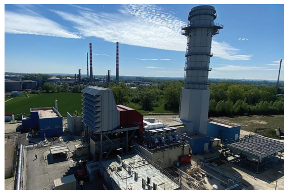
Uniper's Irsching unit 6
