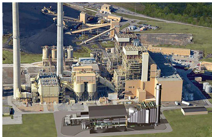
Oklahoma's Grand River Energy Center
