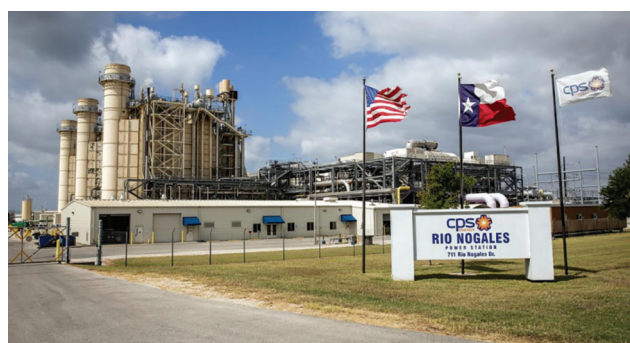
CPS's Rio Nogales gas power plant
