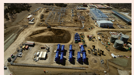
Standing Bear Lake Station during construction
