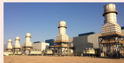
Rumaila power plant near Basra
