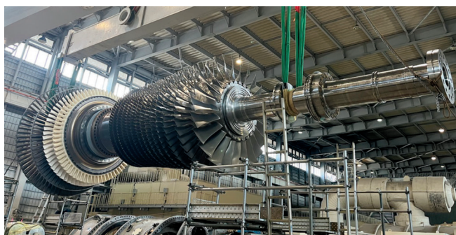
Installation works for the Futtsu 4-3 rotor
