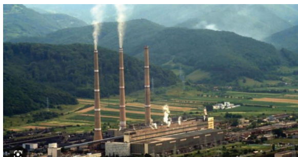
Mintia coal power plant will be replaced by an efficient CCGT
