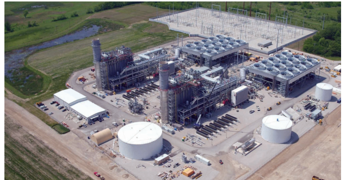
CVP's Three Rivers Energy Center
