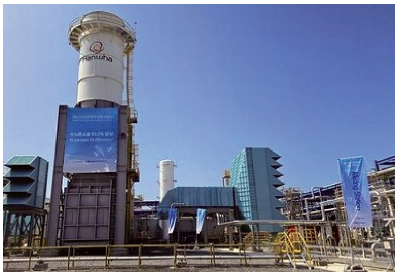
Daesan H2 power plant
