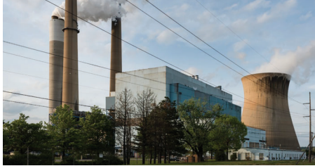
Pleasants Power Station along the Ohio River near Belmont
