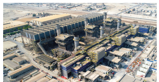
Alba Power Station in Bahrain
