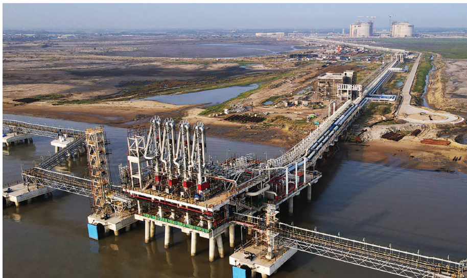
Dhamra LNG terminal at India's east coast
