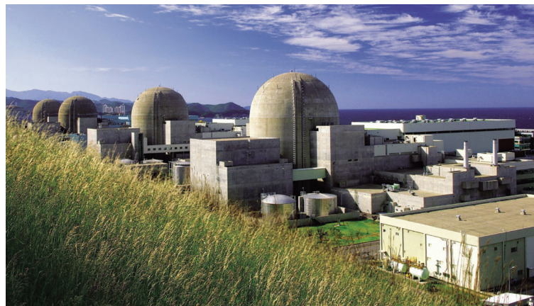
The Hanul nuclear power plant is being extended
