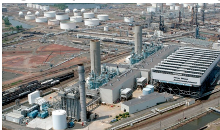
Linden gas power station
