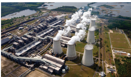
LEAG's lignite-fired plant Jänschwalde was re-instated during the gas crisis
