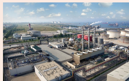
Sembcorp's CHP at Banyan
