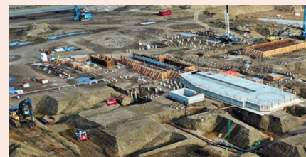
Works at Great Plains power station
