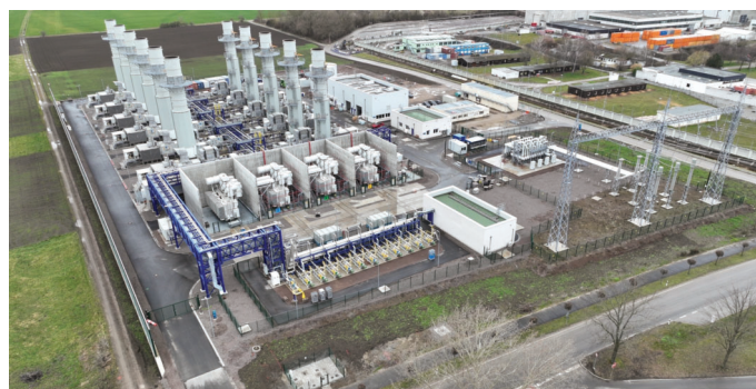
Biblis gas peaking plant
