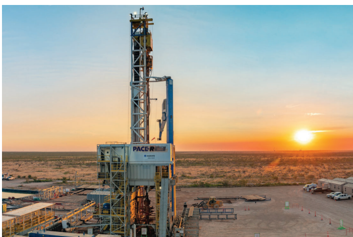
Dry gas drilling rig in the US Midwest
