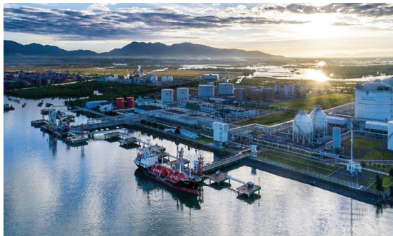
The Thi Vai LNG terminal is almost complete
