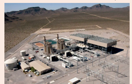
Silverhawk Generating Station
