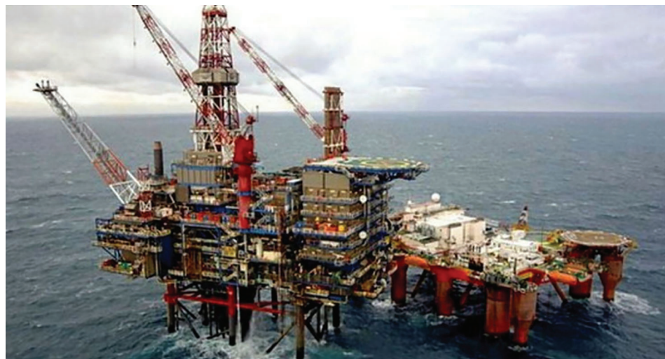
Shell's Nelson platform in UK North Sea
