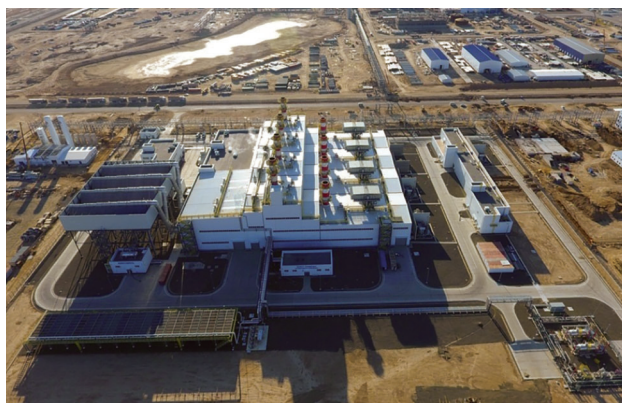
Karabatan CCGT, built by Doosan in 2020
