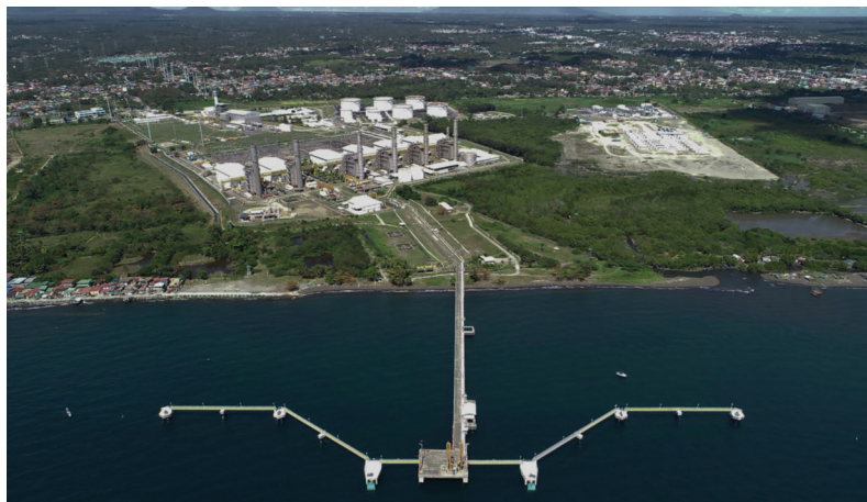
View of BW Batangas regas project
