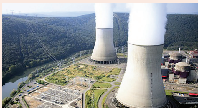
EDF's Chooz nuclear power plant (3.12 GW) in northeast France
