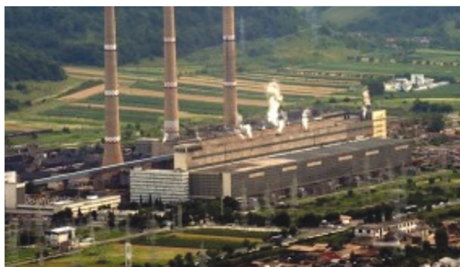
The Mintia coal power plant will be replaced by an efficient CCGT
