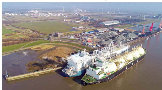
RWE's new FLNG terminal at the port of Brunsbüttel
