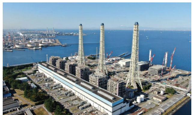
JERA's LNG-fuelled Anegasaki power complex
