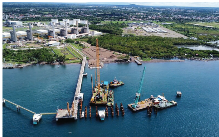
Construction of Linseed's PLNG terminal at Batangas
