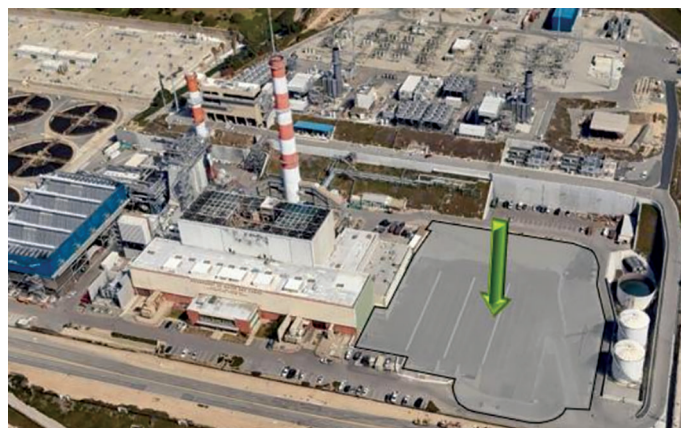
Site of Scattergood repowering project
