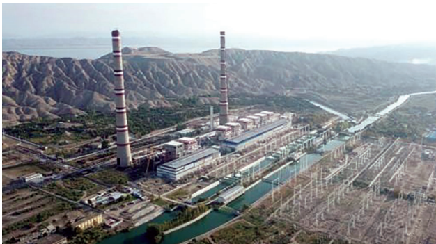
View of the refurbished Mingachevir power station
