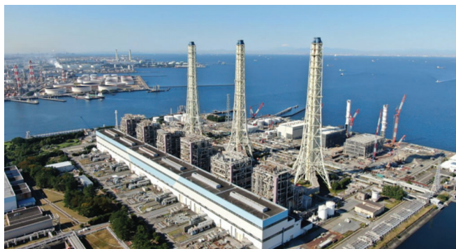
JERA's LNG-fuelled Anegasaki power complex
