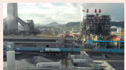
LNG-fuelled decentralised power station in Puerto Rico
