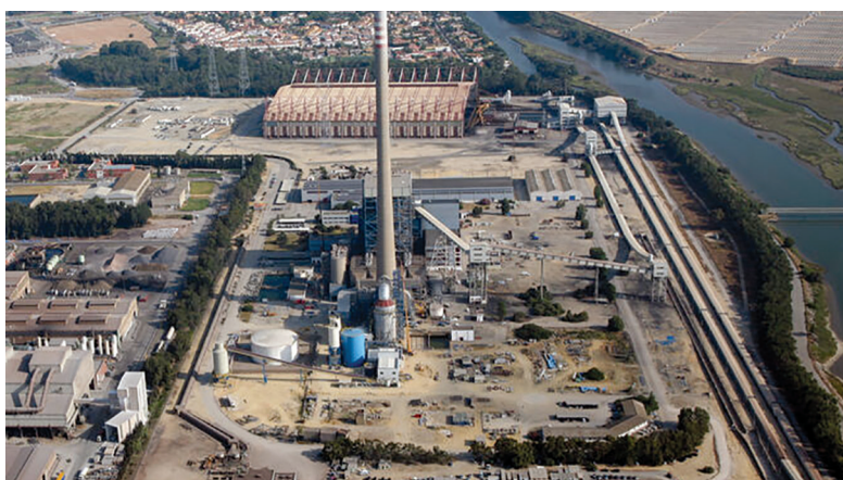
Los Barrios coal power plant (658 MW)
