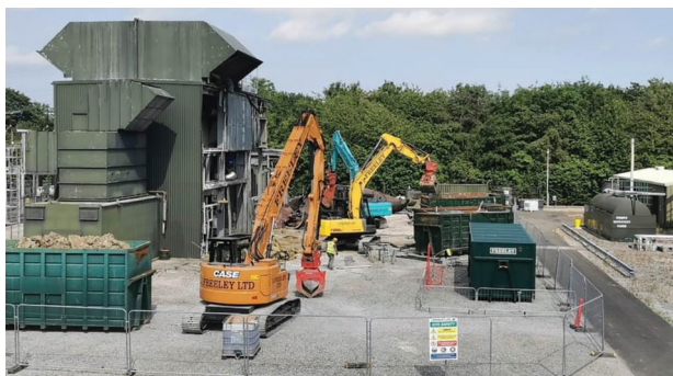
Demolition works at the Knapton site
