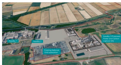
Site of SSE's Keadby power station
