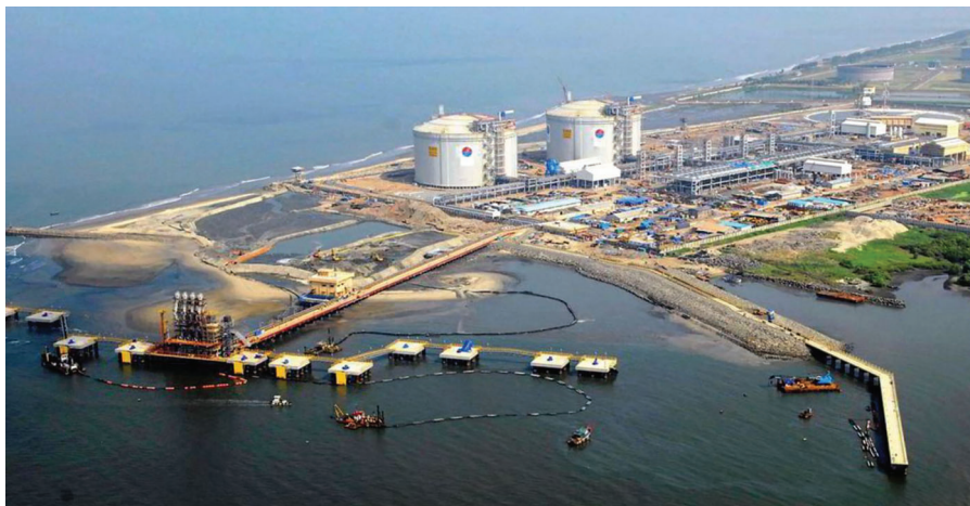
Petronet's Kochi LNG import terminal with a capacity of 5 mtpa
