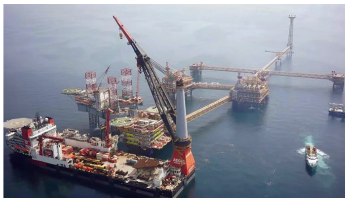
North-Field-platform with Bravo living quarters
