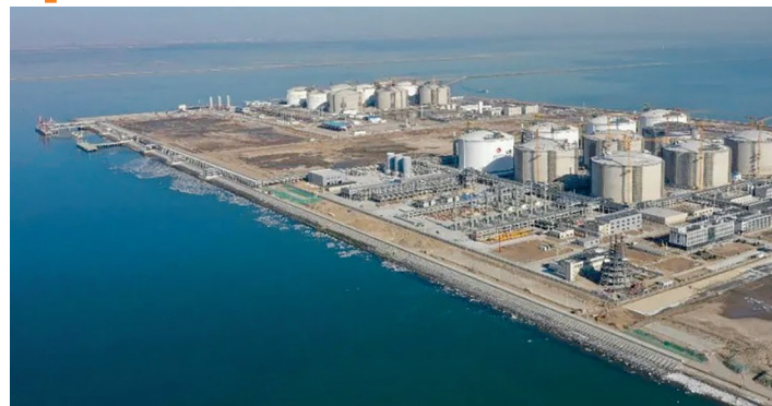
View of Beijing Gas' Tianjin Nangang terminal
