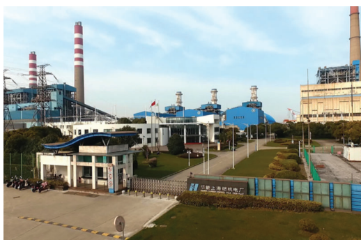
Siemens-built Huaneng Shanghai CCGT
