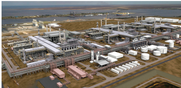
Aerial view of Golden Pass LNG at Sabine Pass, Texas
