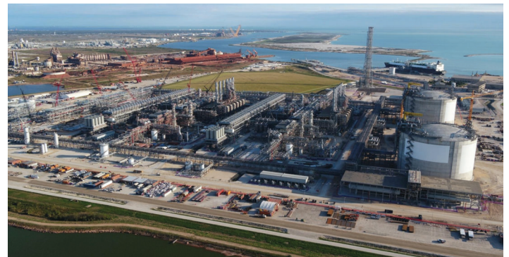
Works progress on Corpus Christi Stage 3
