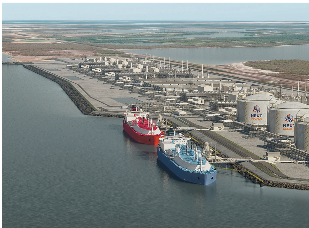
NextDecade has raised cash for Rio Grande LNG Phase 1
