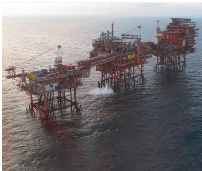
The Rough gas storage facility located off Yorkshire coast
