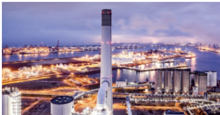
Maasvlakte power hub near the Dutch Gate LNG terminal
