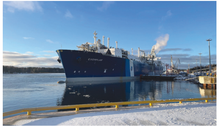
The FSRU 'Exemplar' was deployed in Finland in December
