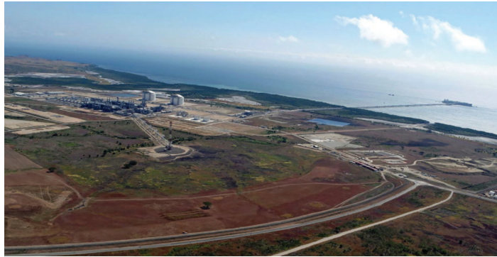
PNG LNG plant at Caution Bay north of Port Moresby
