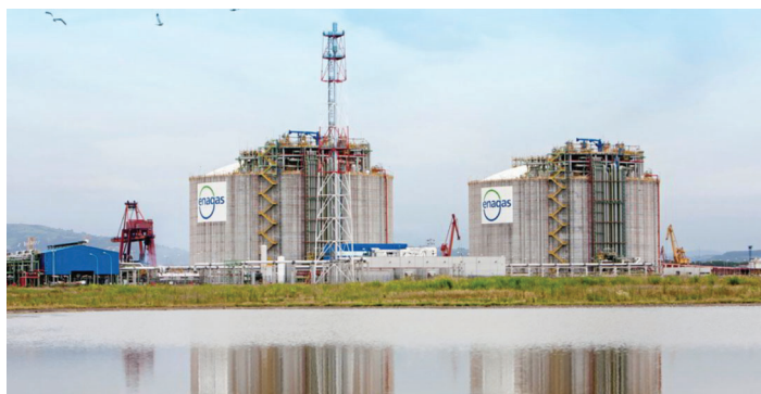
El Musel terminal in the Port of Gijón on Bay of Biscay
