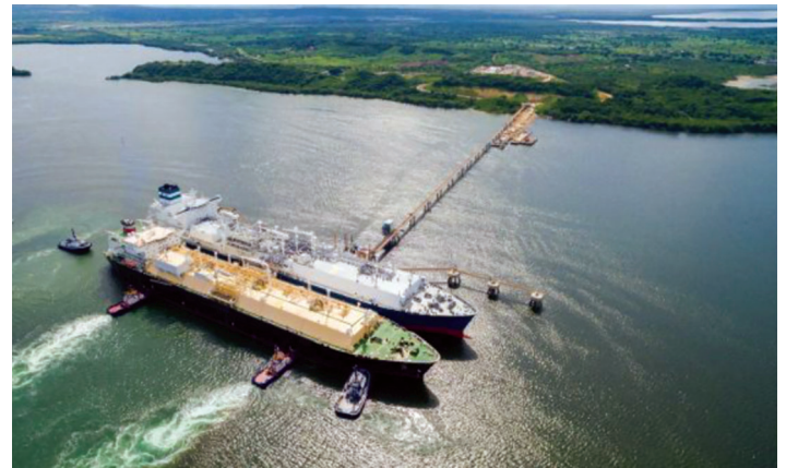
Floating LNG terminal has been at Cartagena since 2016
