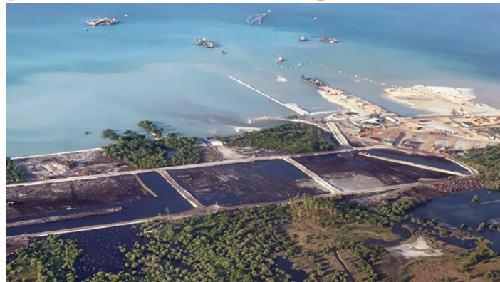
TotalEnergies LNG project site located on Afungi Peninsula
