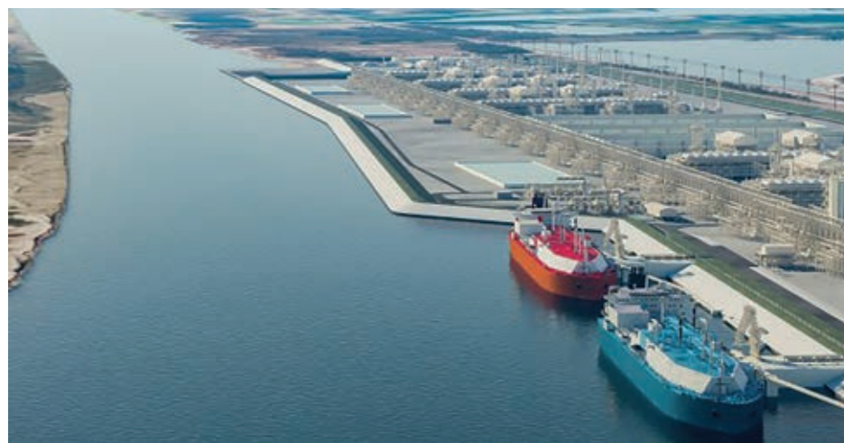
Render of Rio Grande LNG at the Brownsville Ship Channel
