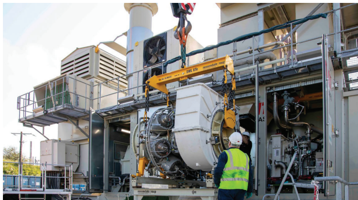
Installation of the SGT-400 gas turbine in Saillat-sur-Vienne
