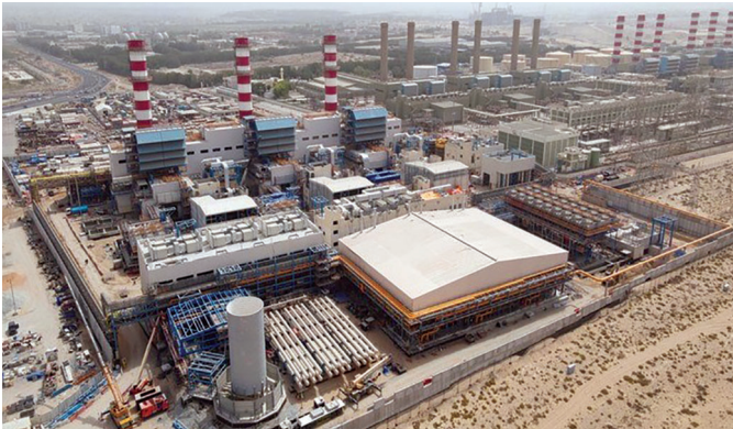
H-Station Phase-4 is 93% complete
