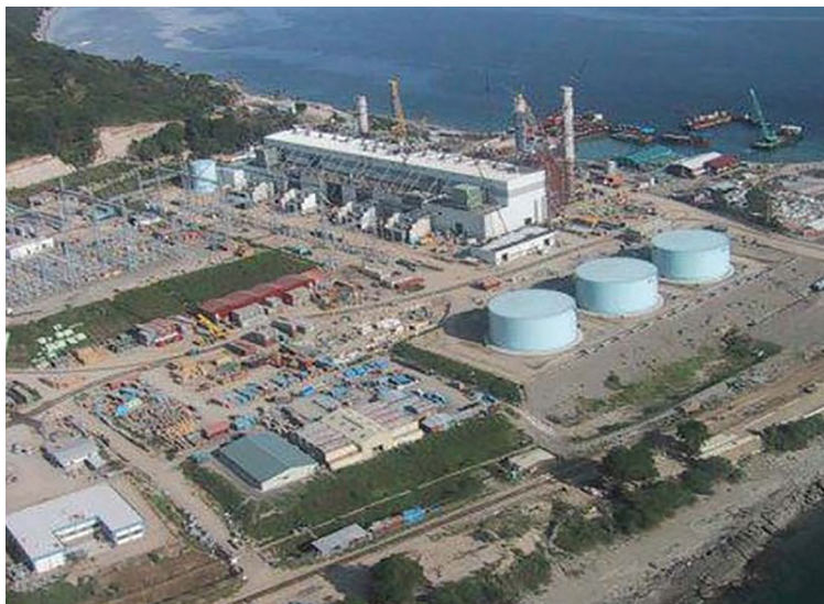
Ilijan power station at a seashore near Batangas City
