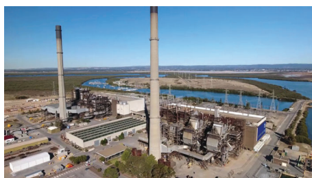
Torrens Island Power Station
